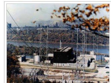
The Shippingport Atomic Power Station in Shippingport, Pennsylvania was the first commercial reactor in the USA and was opened in 1957.
