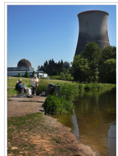
A couple of fishermen near the Trojan Nuclear Power Plant.
